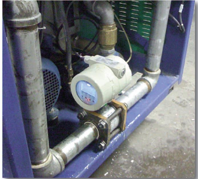
**Model EL 1100 Wafer with MC 608 Electronics
