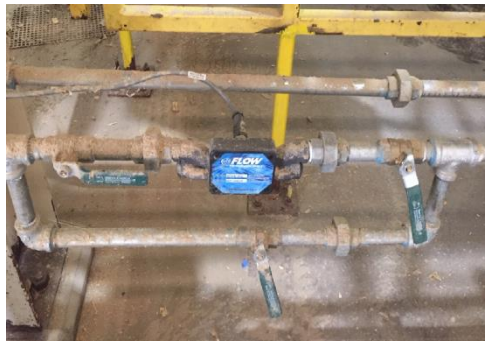
(L) Wood chip dual plate refiner and (R) QCT Series meter at work in a feed line.
