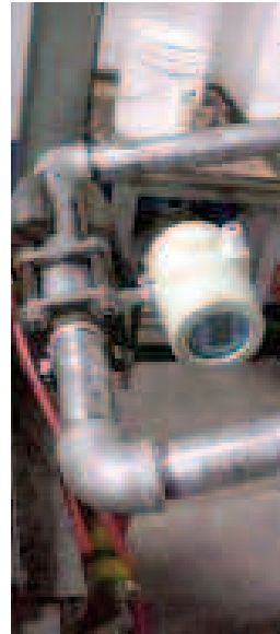
Model EL 1100J Electromagnetic Wafer Flow Meter
